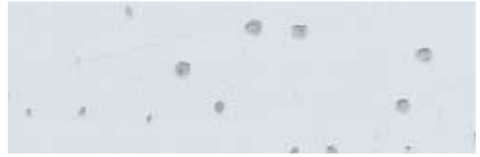
FIGURE 28-11 Pinholes look a lot like chips in the paint.
